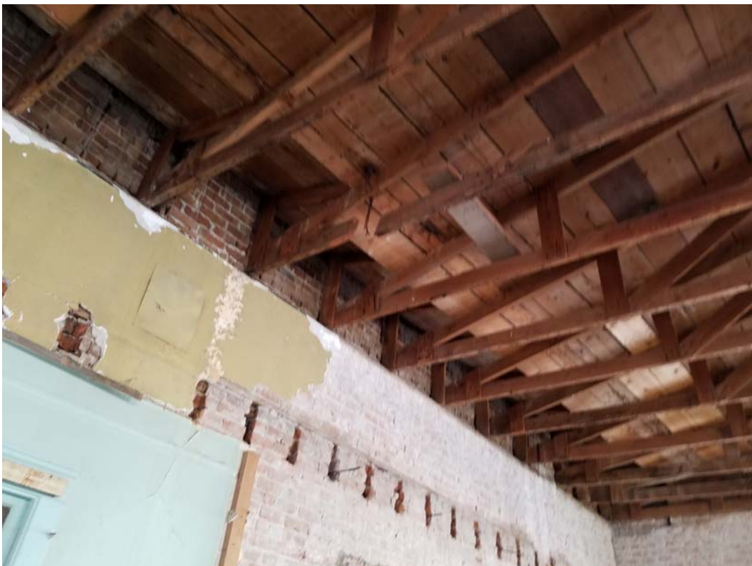
Figure 4 & 5 - Broken Roof Trusses & Original Ceiling Joist Pockets
