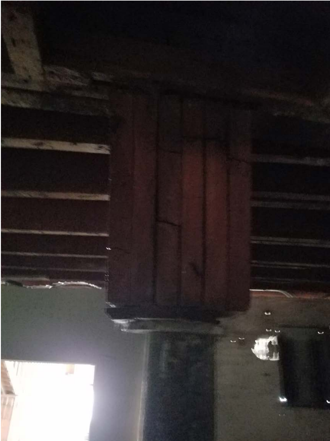
Figure 2 - Built Up Wood Girder and Post Below Second Floor Level
