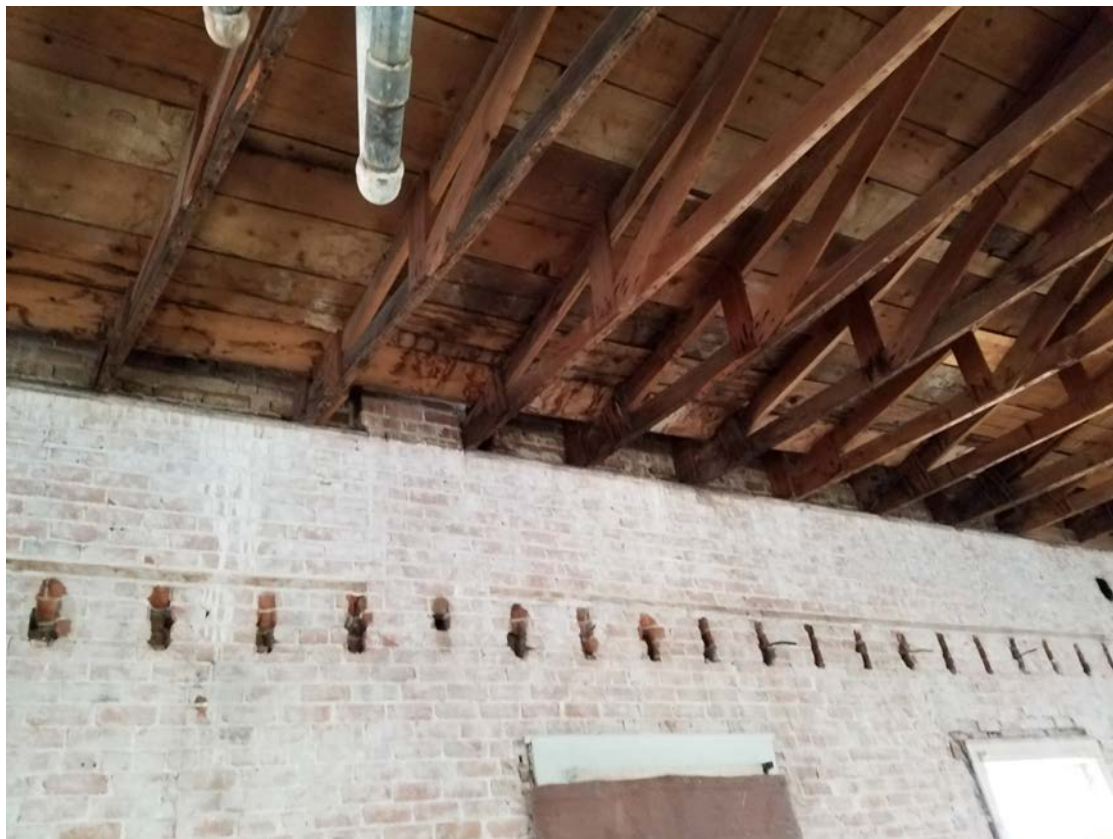
Figure 6 – More Broken Trusses & Original Ceiling Joist Pockets
