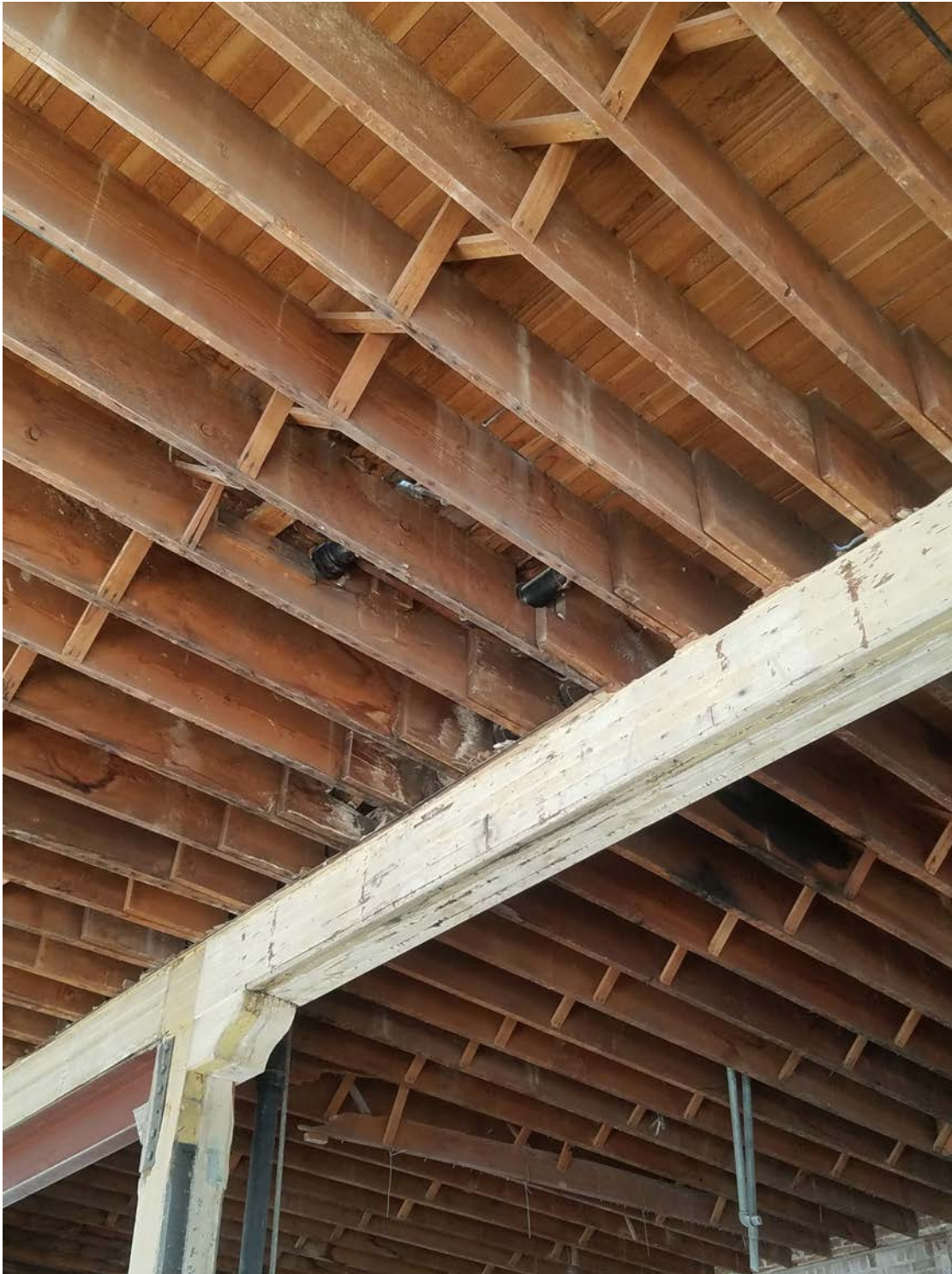
Figure 9 – Second Floor Girder and Broken Joist
