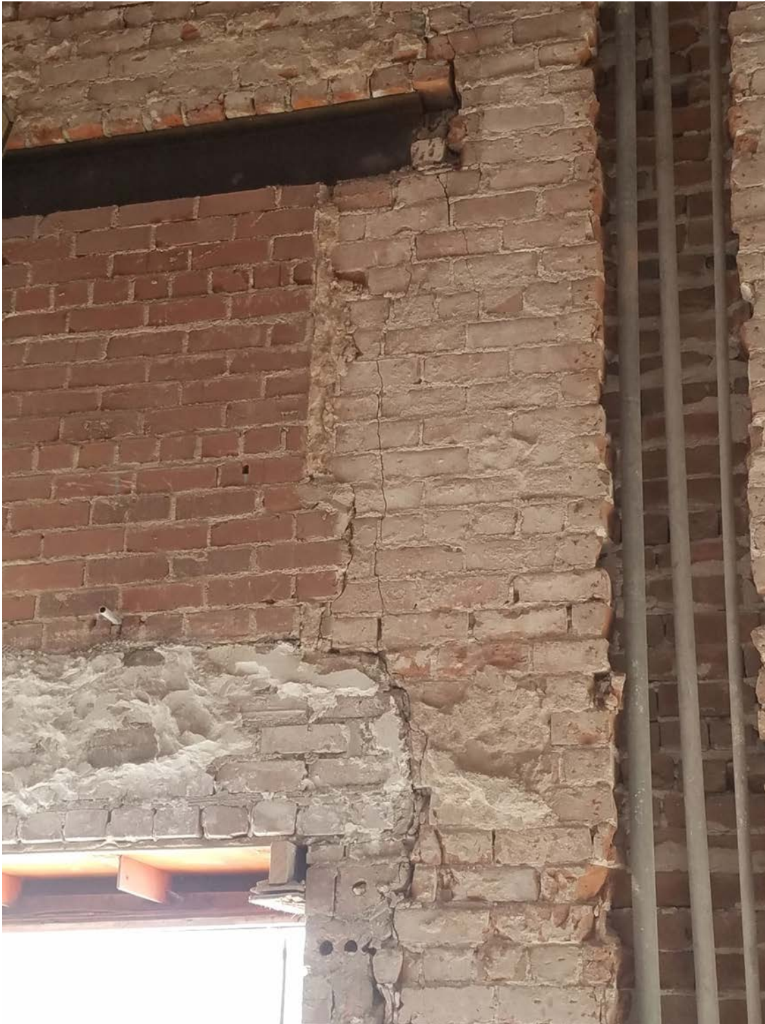
Figure 10 – Vertical Crack at Window Pier
