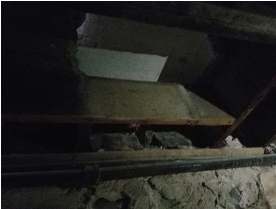
Figure 1 - Stone Rubble Basement Wall and Floor Joists
